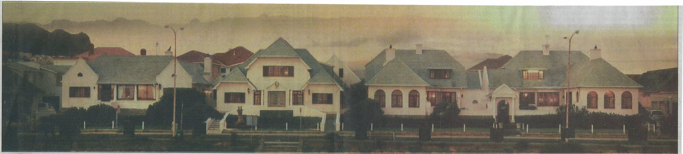
RESTORED: Four Muizenberg beachfront houses designed by Sir Herbert Baker have been linked to create the St Leger Retirement Hotel.
